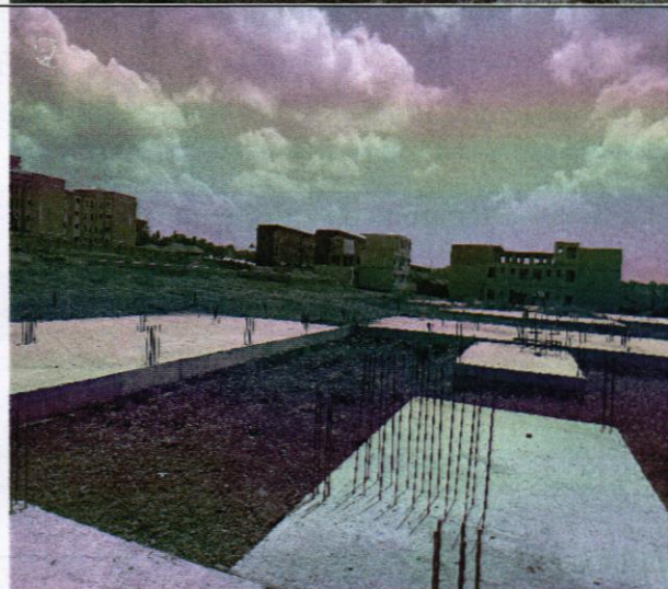
Foundation for Modular Pre-fabricated Housing Units at Naguru
