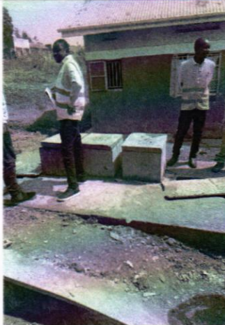
Open septic tank area left without cordoning it off posing risk of injury (left) and poor waste disposal (right)
