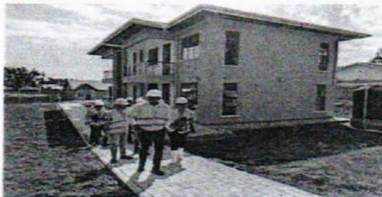
Block of Four 2-bedroom staff accommodation housing units - 99% overall physical progress attained
