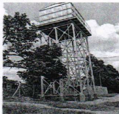
External works (fencing & gates, access roads, landscaping & electro mechanical works - 99% overall physical progress attained Gate house
