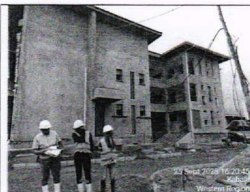
Boys' Dormitory - Double-storey building with a capacity of 100 boys; internal painting was about 80% complete, electrical works were awaiting fittings, and mechanical fittings had been installed. Overall physical progress was at 90%
