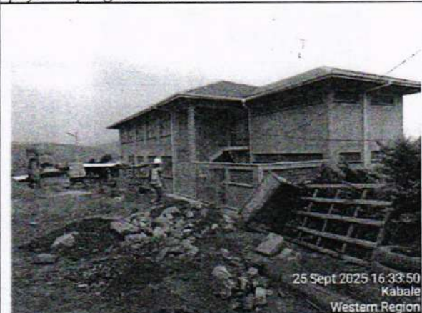
Multipurpose Hall and Kitchen – Started on internal painting - M&E 1 st fix was done – ceiling Works were in progress – Overall Progress was at 50%
