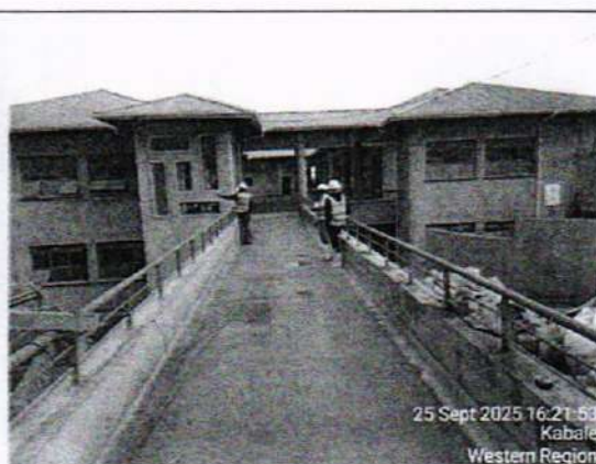
Girls' Dormitory - Double-stored 100 capacity girls' dormitory – comments as above for the Boys' dormitory
