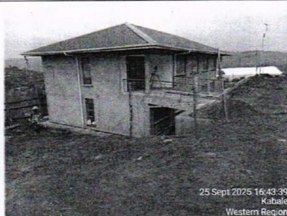
Guard House – Internal plaster was completed – Roof was completed – Overall progress was 30%
