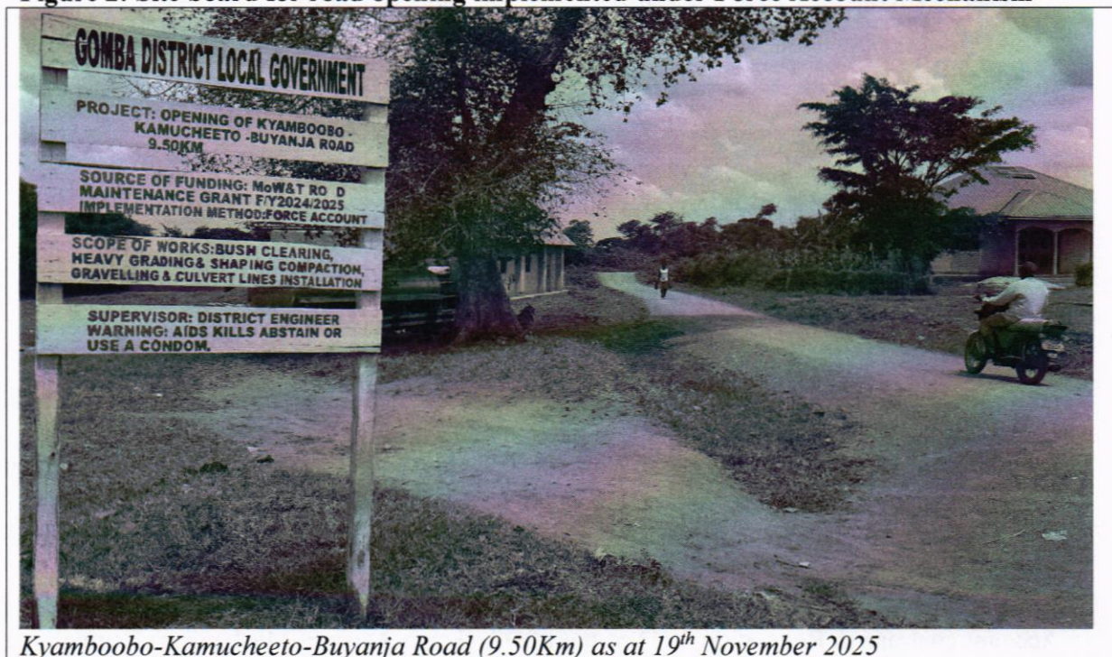
Figure 2: Site board for road opening implemented under Force Account Mechanism
