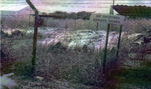
Aviation fuel tanks
