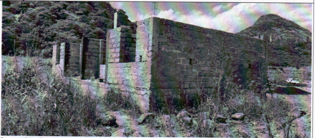
Incomplete Teacher's house 2 as of 17 th June 2026
