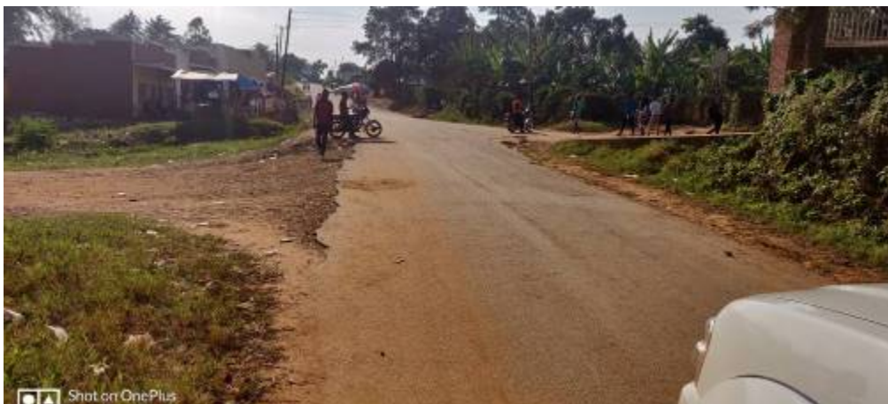
Buremba Road 3.5kms (Maintenance worth UGX 11,258,400) as of 14 th August 2019.
