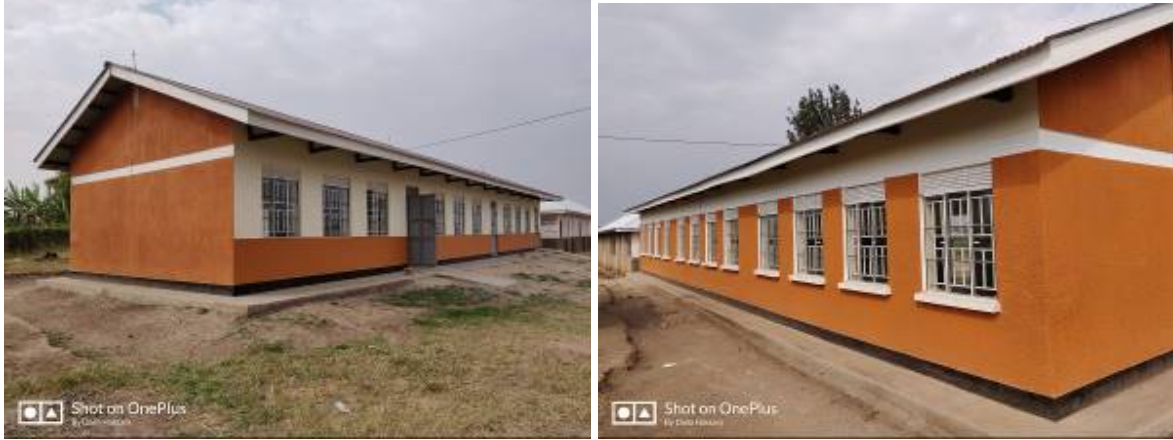
The front and rear sections of the classroom block. Picture taken on 21 st August 2019.
