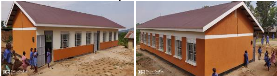
The front and rear sections of the Classroom block. Picture taken on 15 th August 2019.
