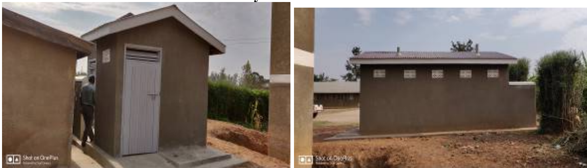
The front and rear sections of the Toilet. Picture taken on 15 th August 2019.
