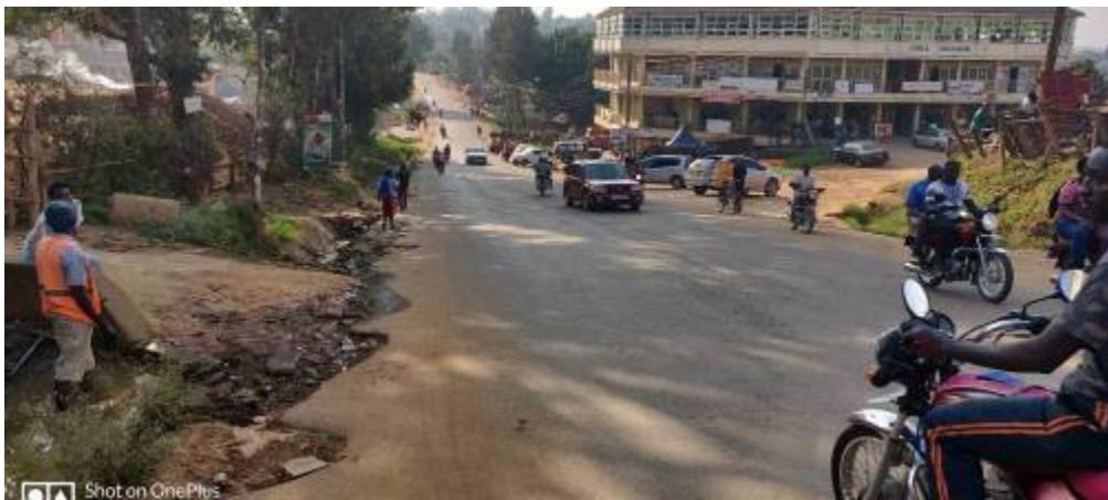
Ntare Road 3.2kms (Maintenance worth UGX 9,938,000) as of 14 th August 2019.
