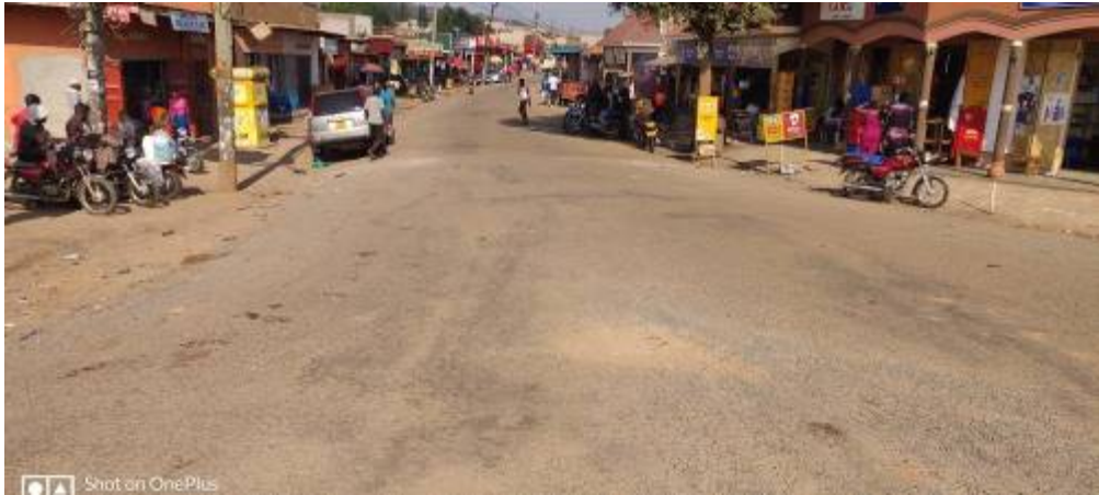
The resealed Koranorya Road (0.5kms) worth UGX 340,802,175 as of 14 th August 2019.
