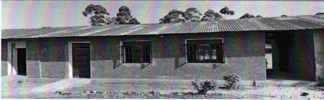
Above: The front view of the completed renovated block
