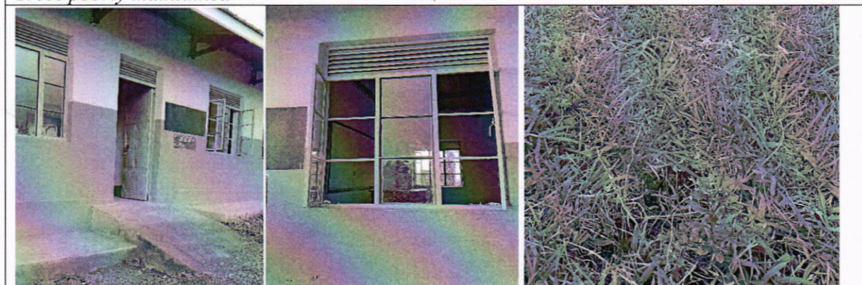
Figure 2: Photo of a steep ramp and cracked floor of a two-classroom block with an office and a store at Kimwanyi Primary School
