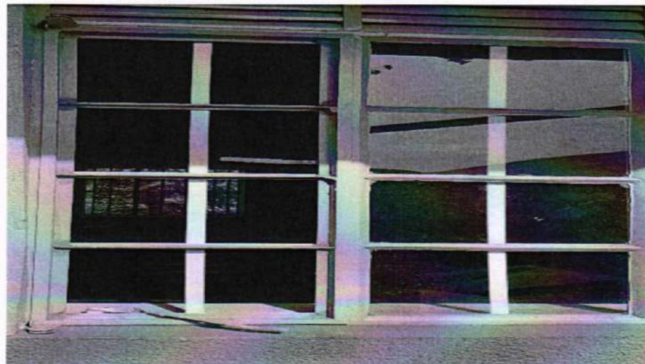
The glasses fell off due to poor mix of patty
