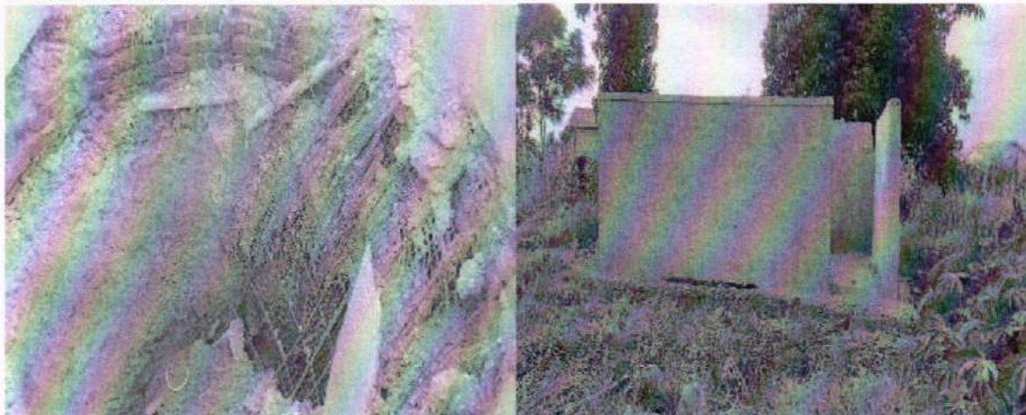
Collapsed/sagged pit
