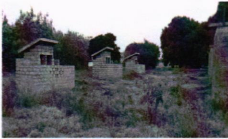
STAFF TOILETS FRONT
