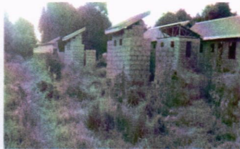
STAFF TOILETS BACK
