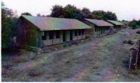
CLASSROOM BLOCKS FRONT
