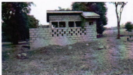
BOYS LATRINE FRONT
