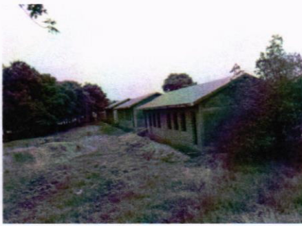
CLASSROOM BLOCK REAR
