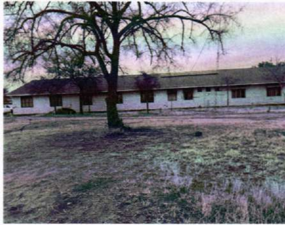
Front view of Health Department Block showing the project site for the renovation works
