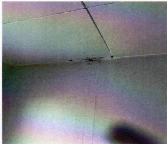
Sections of an interior wall and ceiling corner where water leakage and mold growth are clearly visible.
