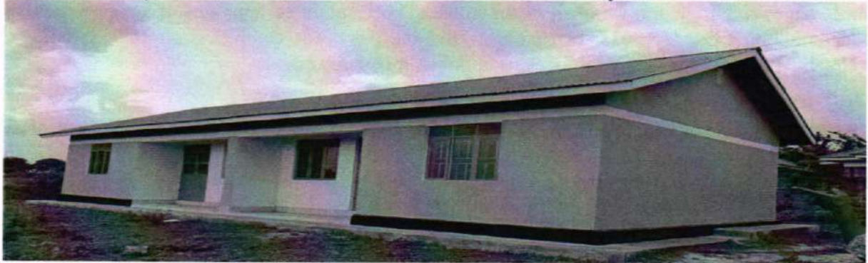
Figure 3: Newly constructed 2-unit staff house at Gisoro Primary School that is not in use
