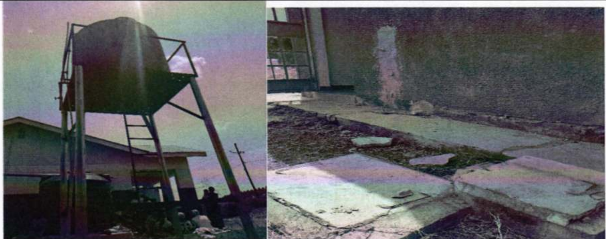
Major crack at the tank base constructed under the contract for the Construction of Staff House at Lucy Bisereko HC III
