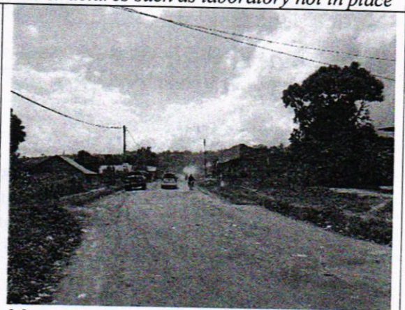
Minor road works
