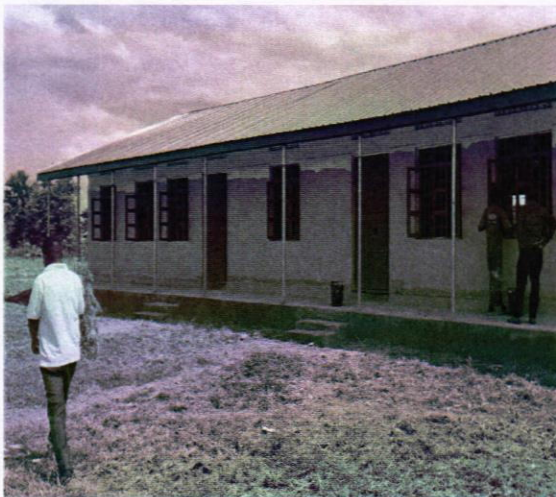
Science Laboratory Block at finishes and painting level
