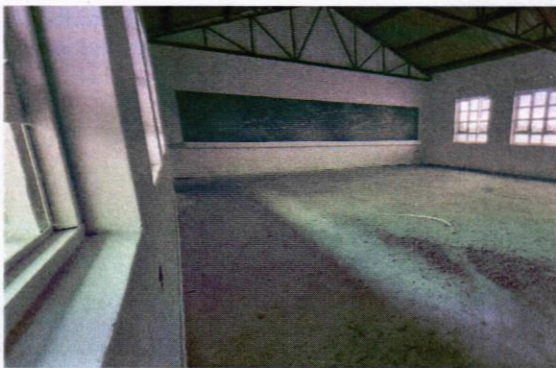
ICT and library Block at final finishes
