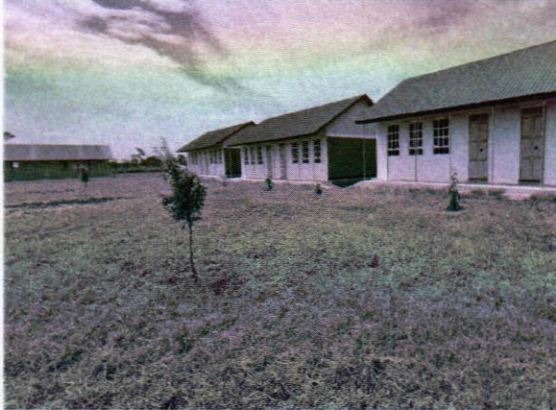
Classroom blocks at final finishes
