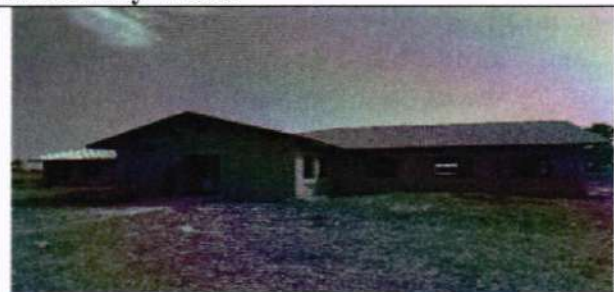
Backview of the incomplete maternity block
