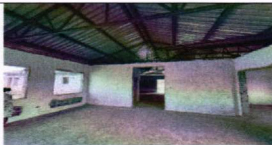
Interior of the incomplete maternity block
