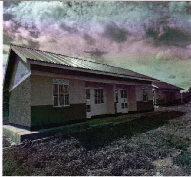
Front view of the staff house
