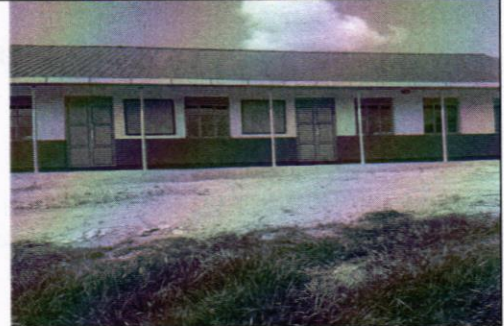
Image 4: Shows the front view of a two class room block
