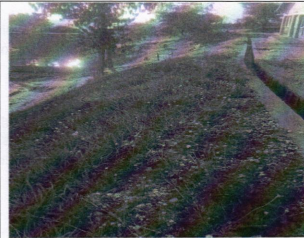
Open drainage channels and grass planting
