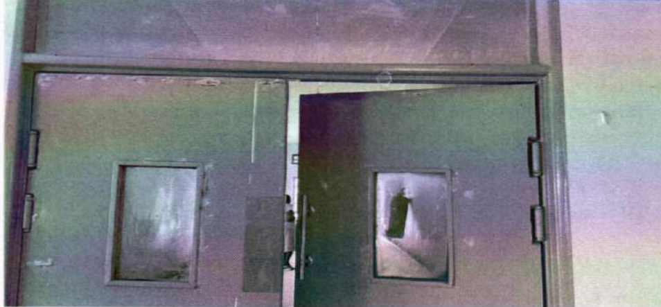
Paint peeling off the doors and the glass were stained and not cleaned
