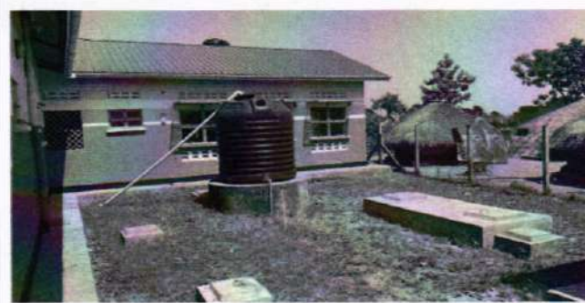
Septic tank and manholes behind Maternity Ward
