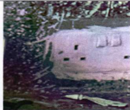
Poorly fixed socket, paint splashes
