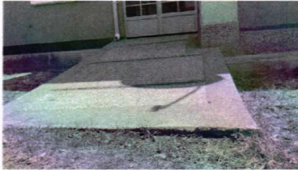
The ramp was not levelled properly with the ground, making it difficult for Persons with Disabilities to move over it smoothly
