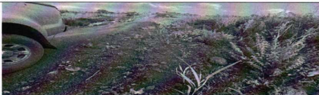
Poorly compacted murram
