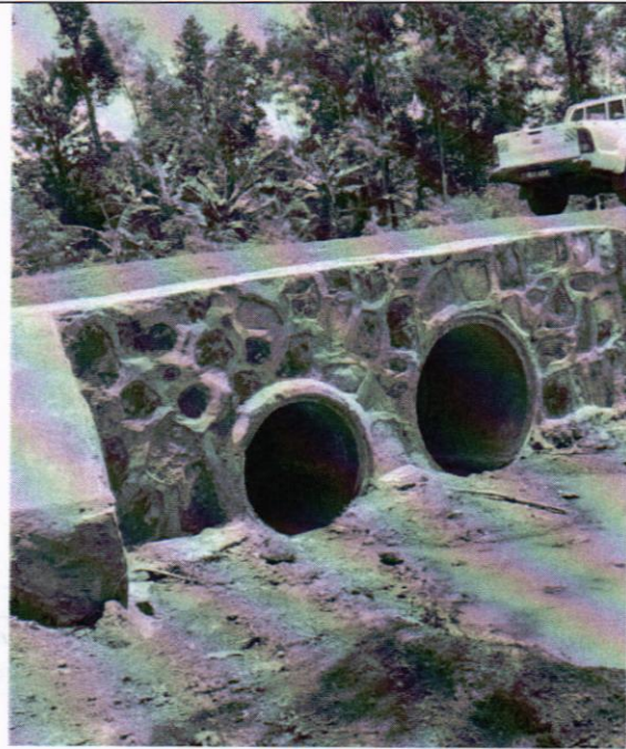
Manakori-Akoret Road drainage wash-away may compromises longevity of the Road and expected to be rectified during DLP
