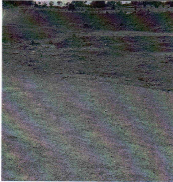
Borrow pit on Makuya-Ndege-Busabi Road not yet restored. Contractor expected to restore borrow pits during DLP
