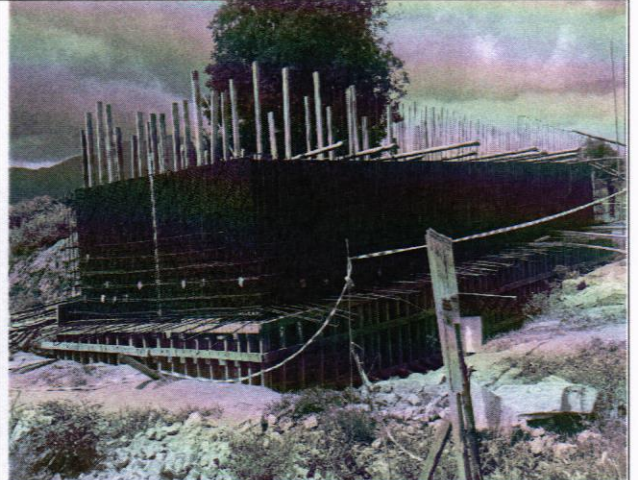
Aerator & sedimentation tank at Laropi WTP
