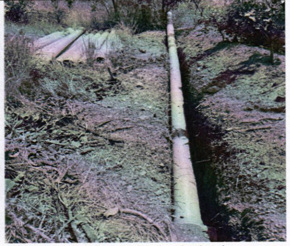
42km Distribution PVC pipe laying in progress
