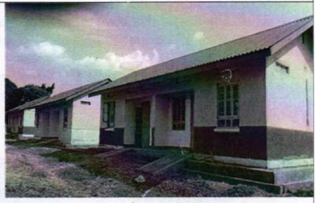
Staff house as of 19 th June 2026; painting works had been completed
