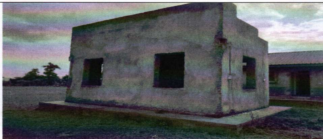
Staff kitchen as of 4 th December 2025, which remained the same as of 19 th June 2026, pending window installation and painting works.
