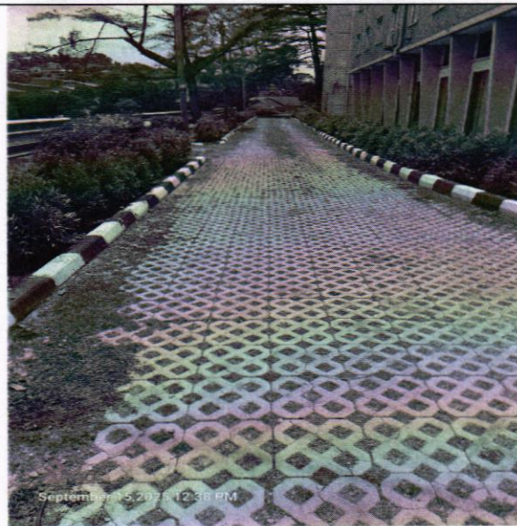
Paved walkway on the upper side of the basketball court
