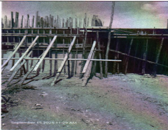
Columns and beams from basement level up to lower ground level
