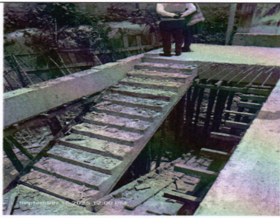
Staircase for the fire escape at the back side of the building
