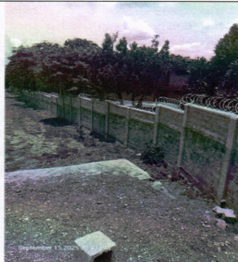
Constructed Parameter wall fence
