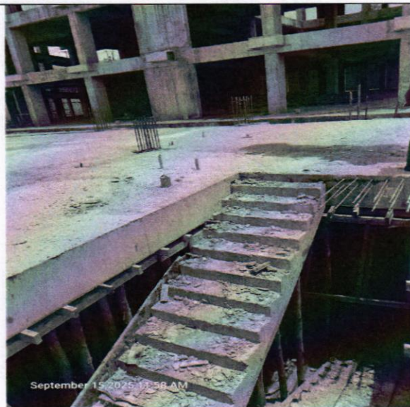
Staircase for the front side of the buliding
