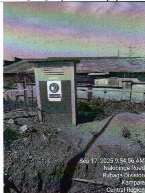
Temporary toilet facility on site
