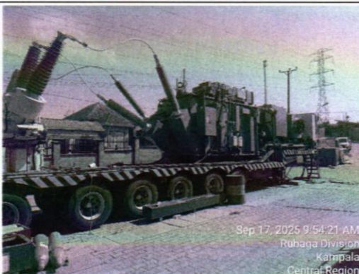
HV Trailer 1 with the power transformer Elevation-1
