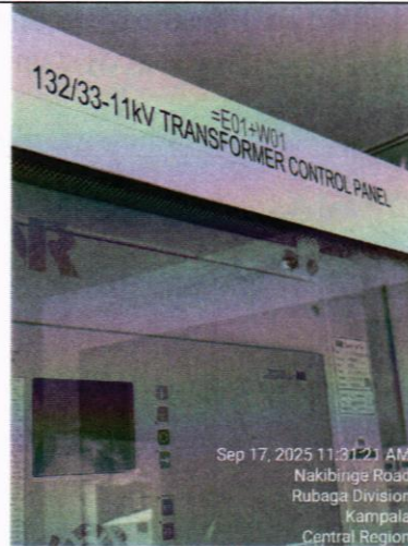
One of the transformer control panels inside the control room
