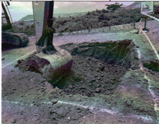
Excavation of transformer location ongoing.
