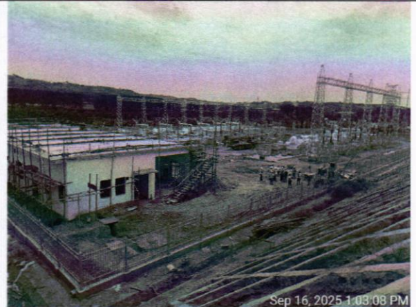
Angled view of the site showing the fence design. It is a steel palisade fence
