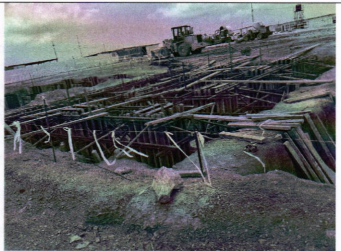
Formwork being set for one of the power transformers.
