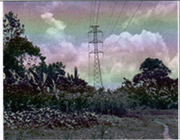
Slanting tower due to effects of vandalism
