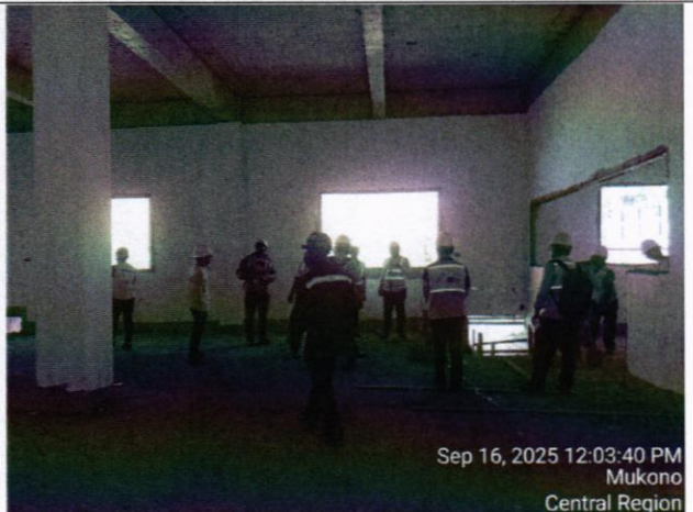
One of the rooms in the control building, the Relay room
