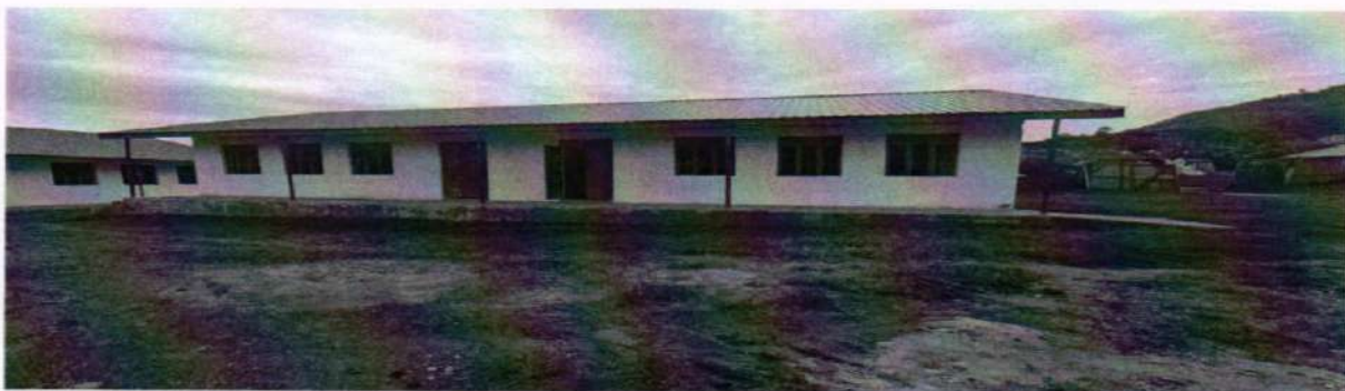
Image 17: shows one of the classroom blocks
