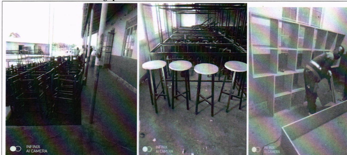
Ongoing works showing the complete frames for ICT hard seat chairs, Laboratory stools and ongoing works on shelves
