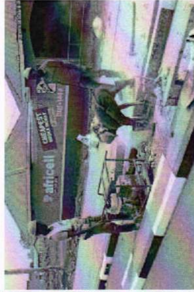
Photographs showing unprotected workers; workers without PPEs such heavy duty gloves, ear plugs and dust masks along Hospital/Chawente Road.
