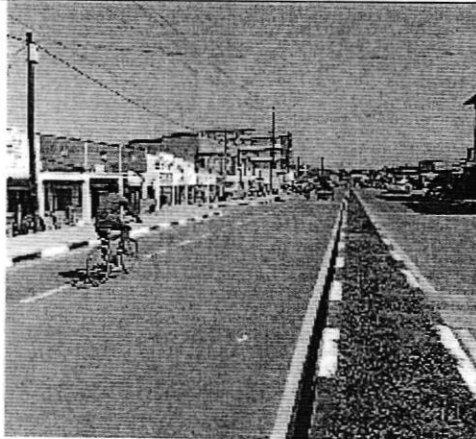
Street lights not yet installed
