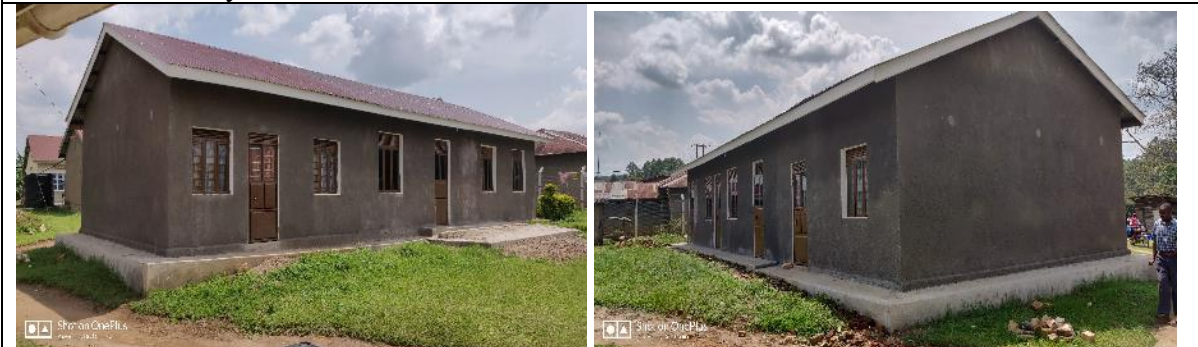
The completed works as of 17 th September 2019
