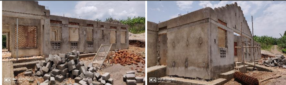
The Health Centre as of 17 th September 2019
