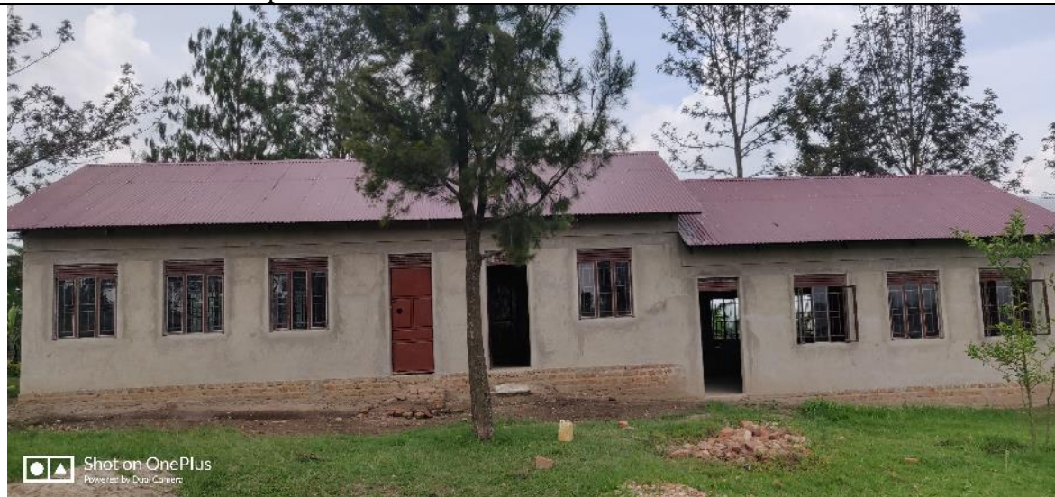
The completed works as of 17 th September 2019
