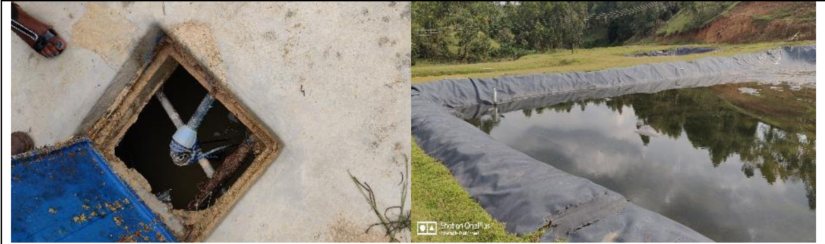
To the left: The shallow well, pipeline and submersible pump. To the right: Ruhandagazi fish fry centre as of 17 th September 2019
