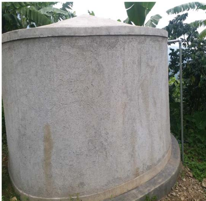
Captioned above is one of the three tanks constructed
