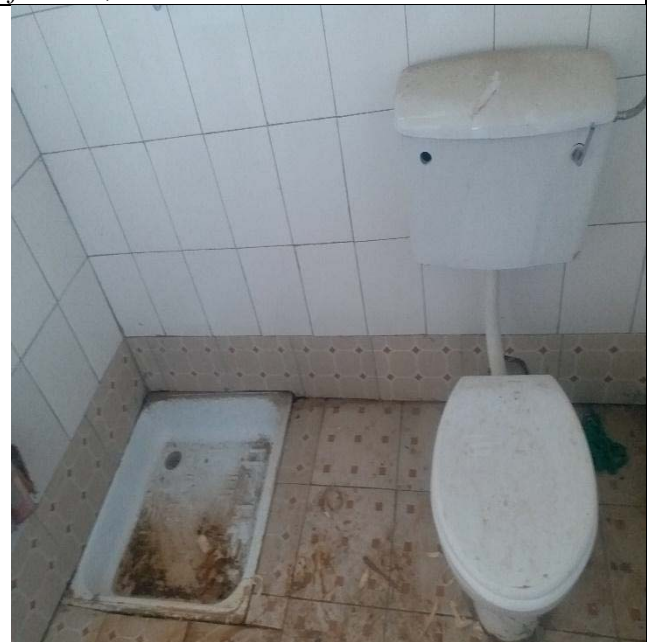
Fixed toilet and bath tub pending connection
