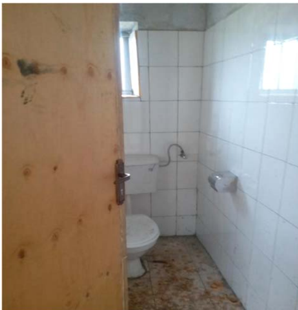
Fixed flush doors pending painting
