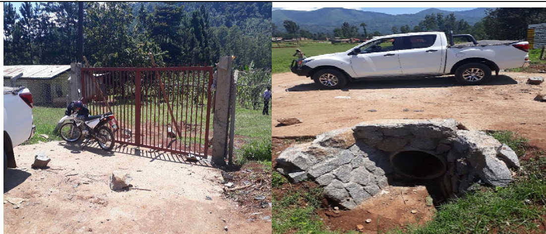
Case 4 & 11: Fencing of District Natural Resources and Production Office Land
