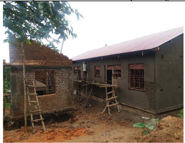
Two Unit staff houses at plaster level
