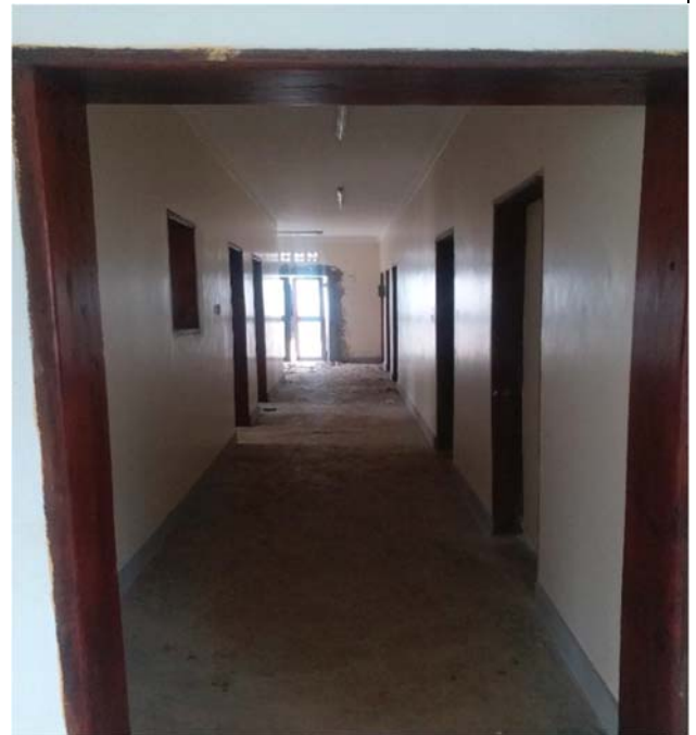
Interior works including painting, fixed door frames , electrical works
