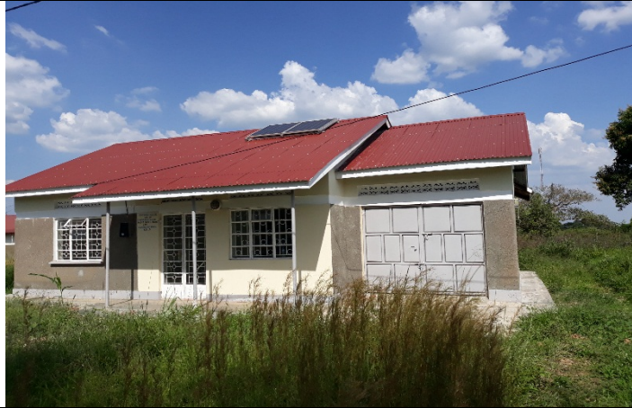
Rehabilitated Doctor's House at Tirir HC IV
