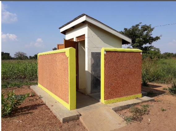
Completed Pit Latrine at the Teachers House at Ojago Primary School
