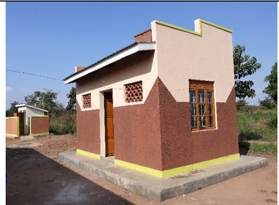
Completed Kitchen at the Teachers House at Ojago Primary School
