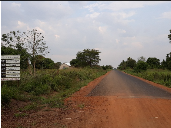
Low cost sealing of Kamuda-Aboket Road phase three (0.4 km) – RTI
