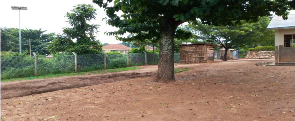
Image 7: Completion of chain-link fencing at Nabuyonga Primary School
