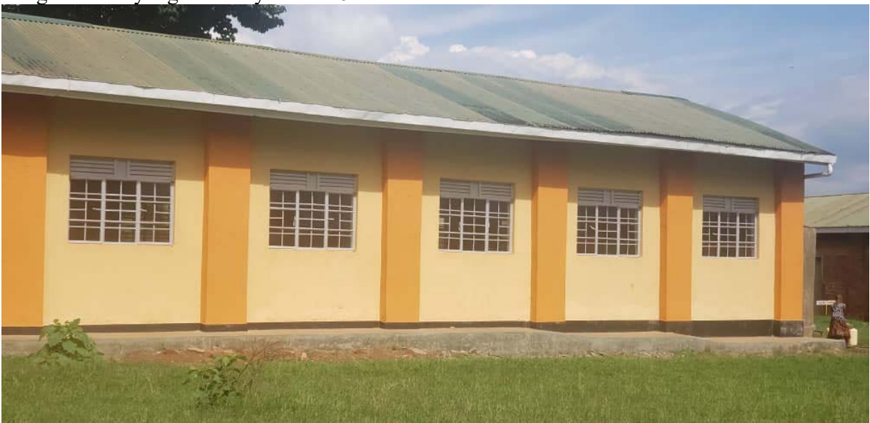
Image 5: Renovated two classroom block at Wambwa Primary School
