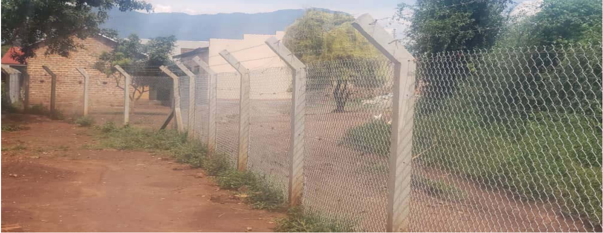
Image 6: A section of a chain link fence at Doko Primary School
