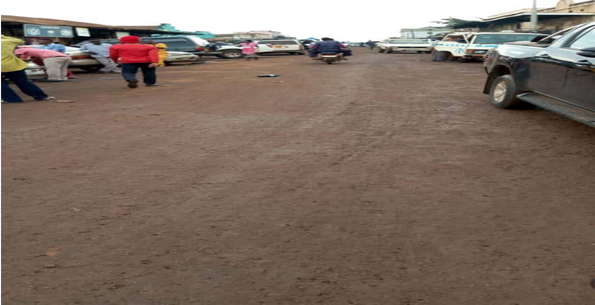
Image 1: Low cost sealing of 250 meters of Maluku road under force accounts
