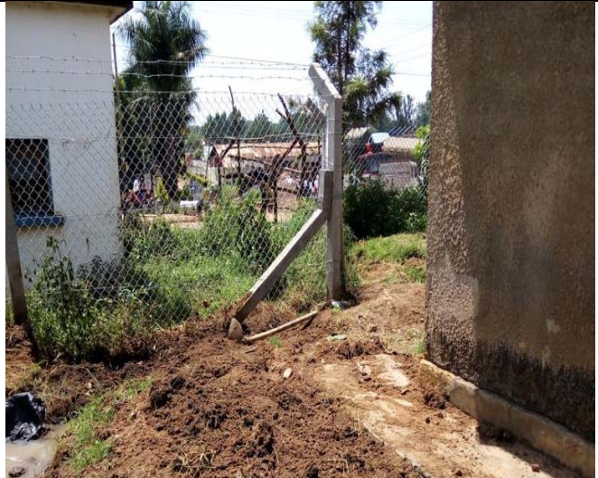
The defects on the fence at Mbale Police Wanyera were rectified.
