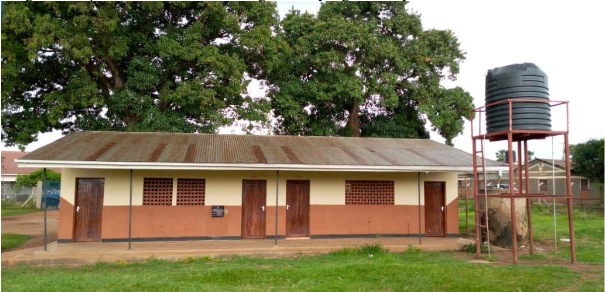
Image 8: Rehabilitated water borne toilet at Namakwekwe Primary School
