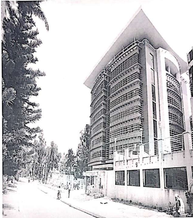
A picture of the PPDA/URF Project progress
