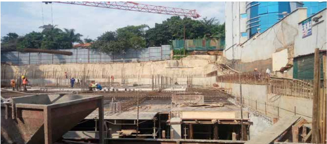
Preparation of maxpan slab on the ground floor level(27/06/2019)
