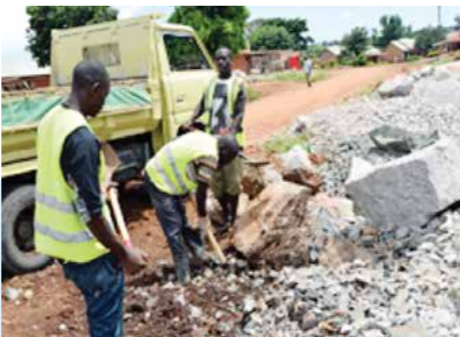
Construction of Busia-Majanji Road
