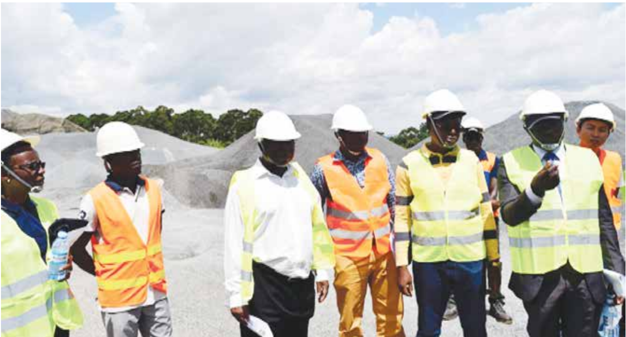
PPDA team conducting on spot verification on construction works of Musita-Lumino and Busia-Majanji Road and Rehabilitation of Nakalama-Tirinyi Roads
