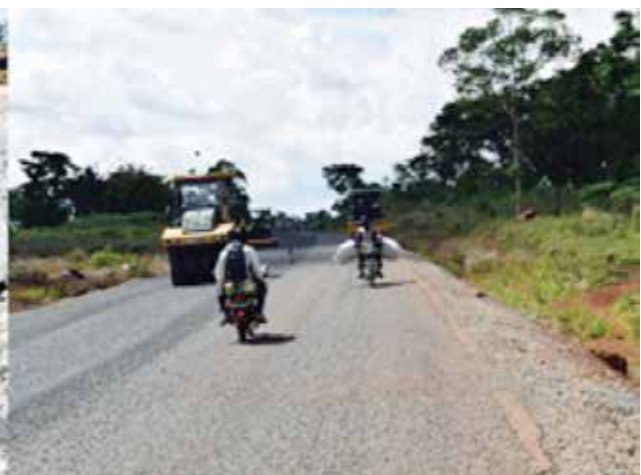
Construction of Nakalama-Tirinyi Road
