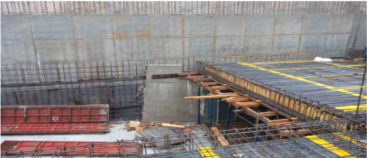
Ground floor rebar works at extent to receive generators (13/06/2019)
