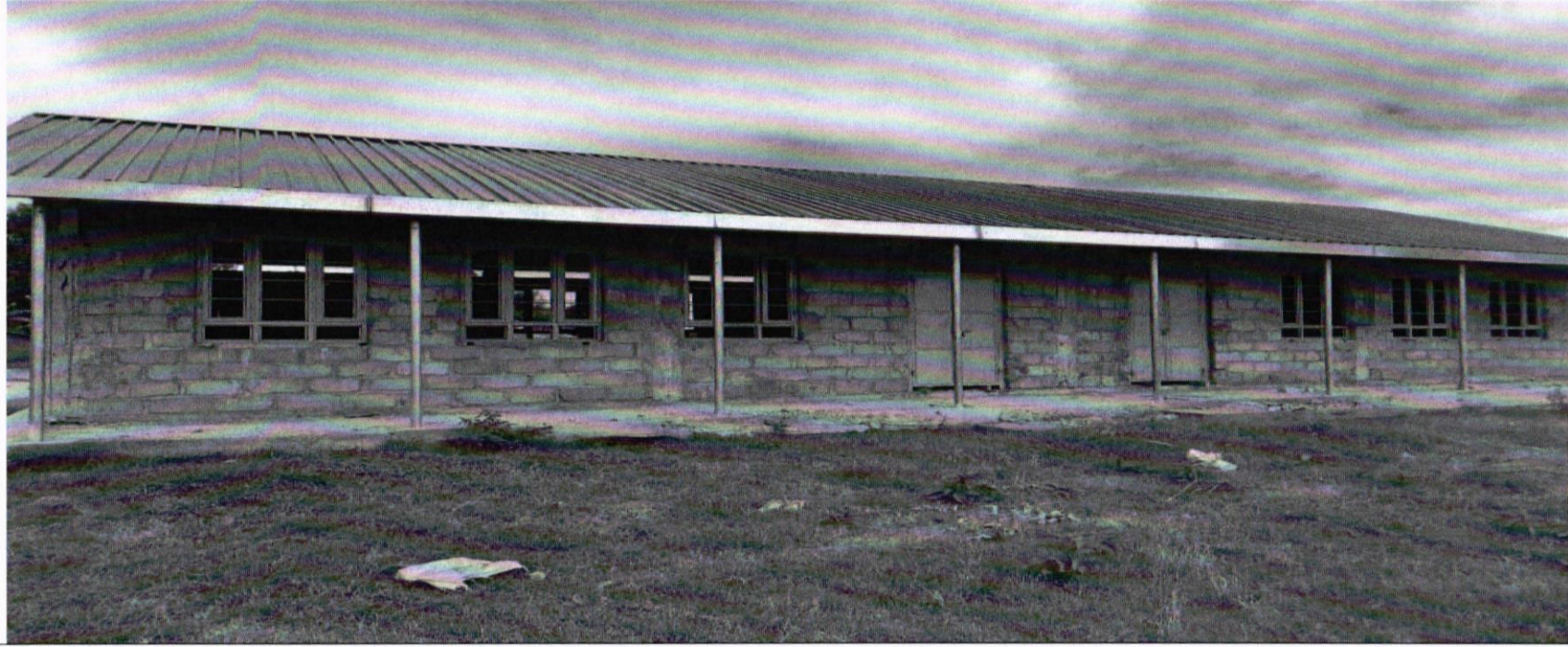
Administration block Moyok
