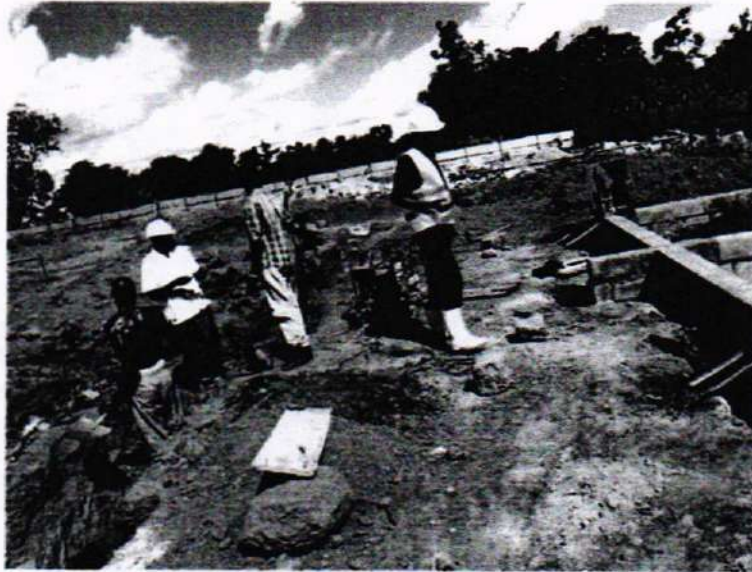
Pictorial showing the nature of the hard surface and the equipment used to excavate.
