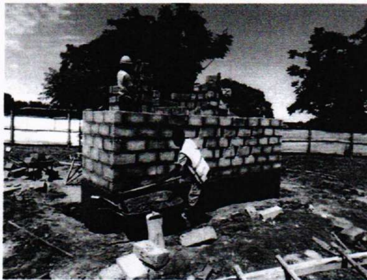
Pictorial showing ongoing construction works on a 2 stance drainable pit.
