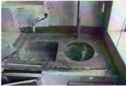
Poor finishes, incomplete sinks and one of the pinboard with brown staining, respectively.
