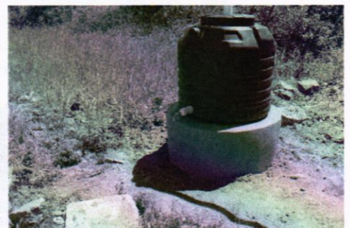
Unpaved, uneven soil and bushy site obstructing access to the Male toilet, missing armrests or grab rails; and 500-liter overhead tank without a soak pit, respectively
