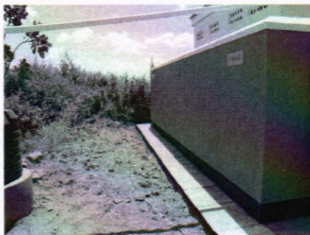
Unpaved, uneven soil and bushy site obstructing access to the Male toilet, missing armrests or grab rails; and 500-liter overhead tank without a soak pit, respectively
