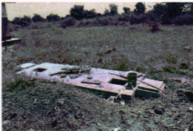
Absence of safety signage, warning tapes around dangerous spots like the open septic tank and broken glass, and the site was unfenced (not hoarded), unlit, unguarded and overgrown with a bush.
