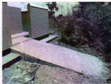
Inaccessible ramps to both the Female and Male toilets respectively
