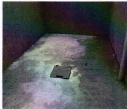
Poor paint finishes inside and outside the placenta pit and the jammed door, respectively
