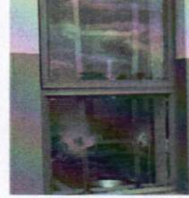
Windows where the stays and fasteners were welded
