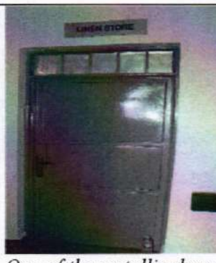
One of the metallic doors installed at the Linen Store
