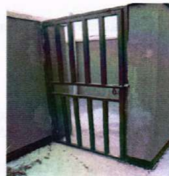
Poor paint finishes inside and outside the placenta pit and the jammed door, respectively
