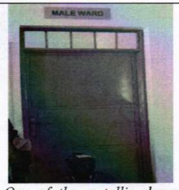
One of the metallic doors installed at the Male Ward
