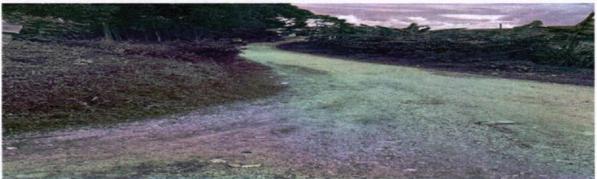
Image 6 shows a section of Butare Kajugangoma Road as of 27 th March 2025
