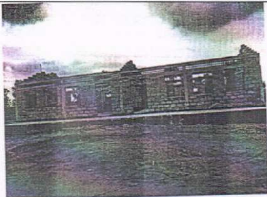
Figure 4: Shows the laying of air bricks for ventilations in two classroom blocks.
