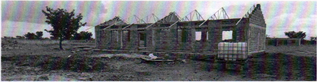
Classroom Block 2 at roofing level
