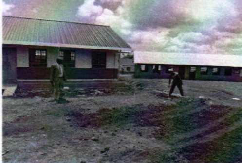
Compound levelling works ongoing
