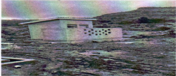
2 stance lined pit latrine for the admin block.
