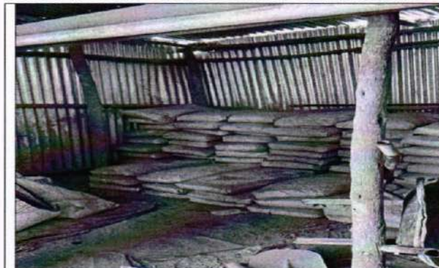
Cement in store but the store has no doors to protect against theft and harsh weather
