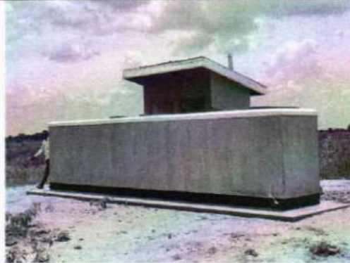
Front view of two stances pit latrine
