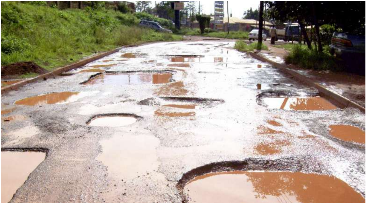
Potholes are caused by shoddy work that reduces the quality and life span of roads
