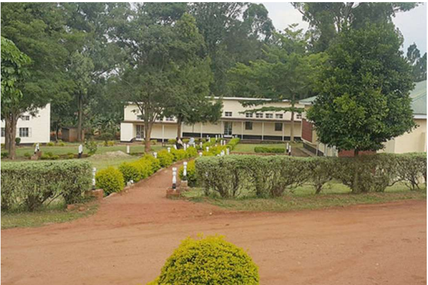
Classroom blocks at Bukalasa College. Budget allocation funds were released for running the college during Covid times even though it was closed due to the lockdown
