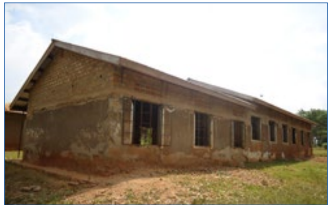
The Ndwadde Mutuwe Primary School classroom block
