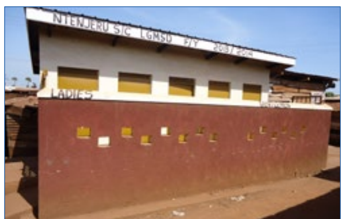
Toilets in Kisoga trading centre, Mukono, built but never used
